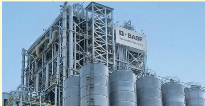
loopamid’s plant in Shanghai
